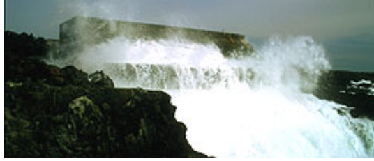
The Limpet-plant in Islay
